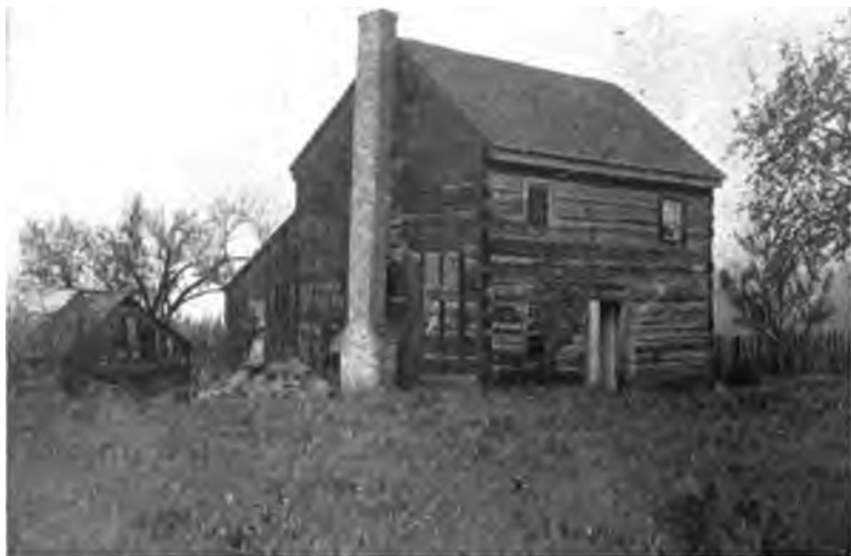
House Built By William Ewing, at Ewington, Ohio, 1812.
